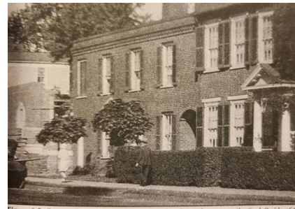
Figure 6-2. Construction of University Baptist Church can be seen on the far left side of the picture of the Upper Main Street Building (Library, University of Virginia)
